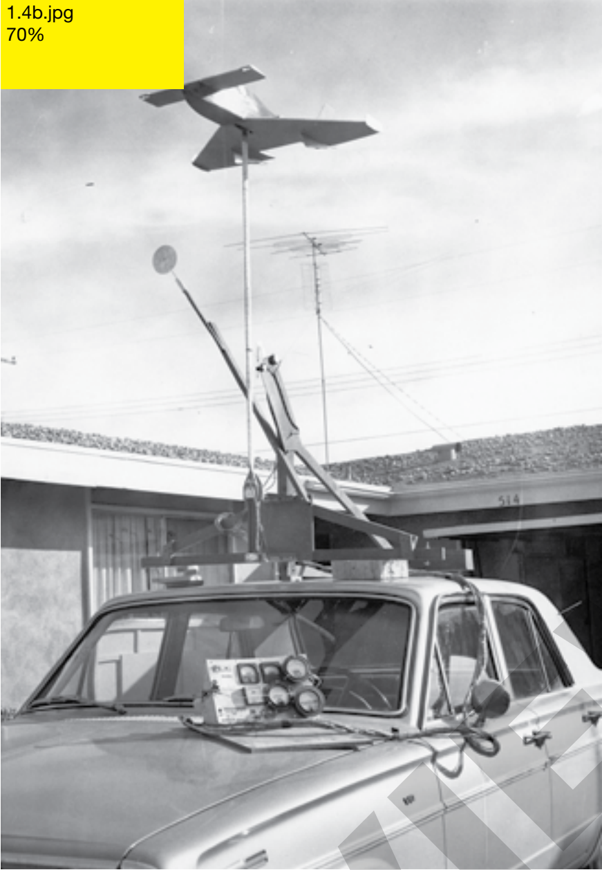
Burt Rutan created his own wind tunnel, and as long as the pavement didn’t run out, there was plenty of wind to test his designs. By attaching a model to an array of sensors mounted on top of the family car, he was able to collect flight data from a set of instruments as he sat in the passenger seat. Courtesy of Burt Rutan
