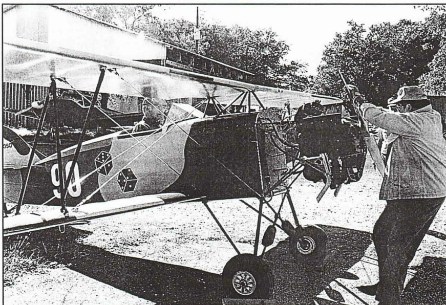
Turning the prop through four or five blades before attempting to start the engine each day will give you a number of important cues as to the condition of your engine. How many can you think of? Refer to the text under "Engine Starts."
