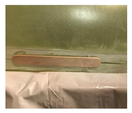
I actually ran the Zap-A-Gap around the edges of the stir stick and sprayed it with accelerator and pushed it onto the two edges bringing them into alignment for the length of the stir stick. Note the edges don't always touch...
