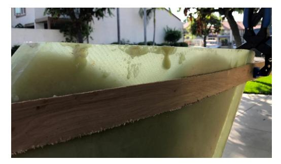
So I mixed up a 1/4 cup part A&B and mixed that up and poured it into the top - but it came up short, so I mixed up another  $\frac{1}{4}$  cup and found the foam topping out the pylon so I used the mixing cup to scoop up some of the unnecessary foam and slide it to other parts of the pylon top.
