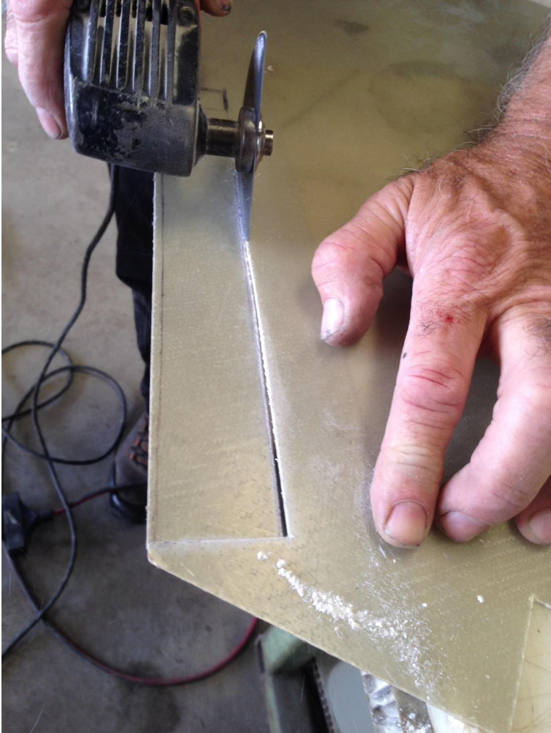
21. Cutting the faux elevator bottom skin off scrap glass.
