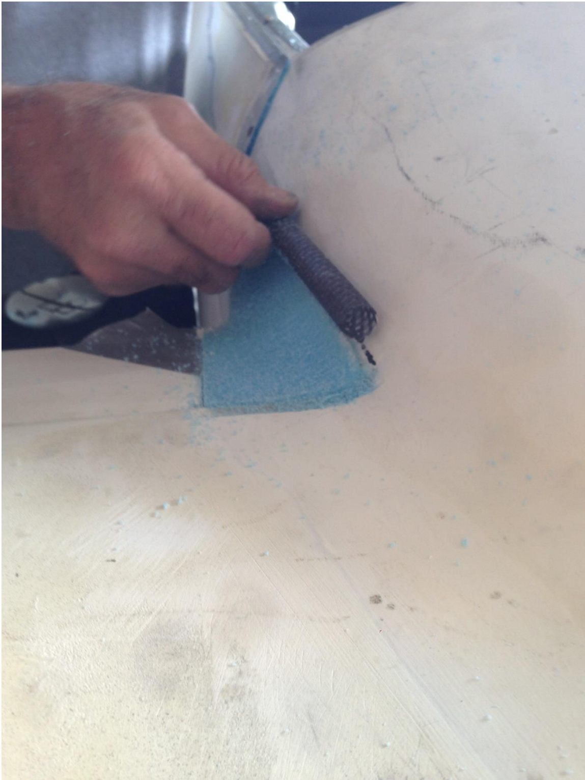
27. Right side trimming for glass.
