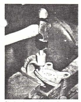
Riveting the new lining to the pressure plate calls for 10 to 20 medium blows from a 10-ounce ball-peen hammer. The assembly should be rotated from side to side while hammering, to clinch the rivet head evenly.
