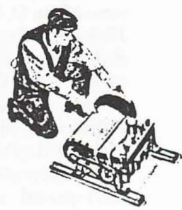
At 12 horsepower, the Wrights' aluminum four-cylinder, water-cooled engine was the first to lift a craft into the air age.
